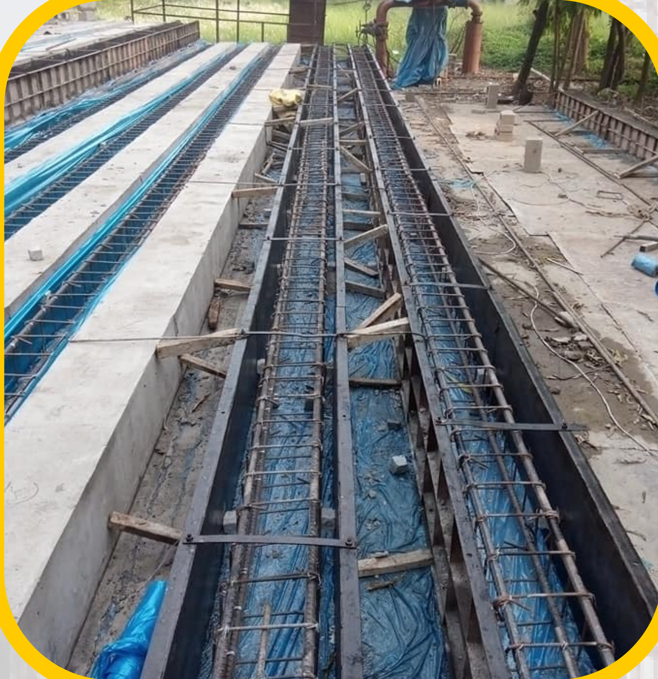
Pre Cast Pile Making
