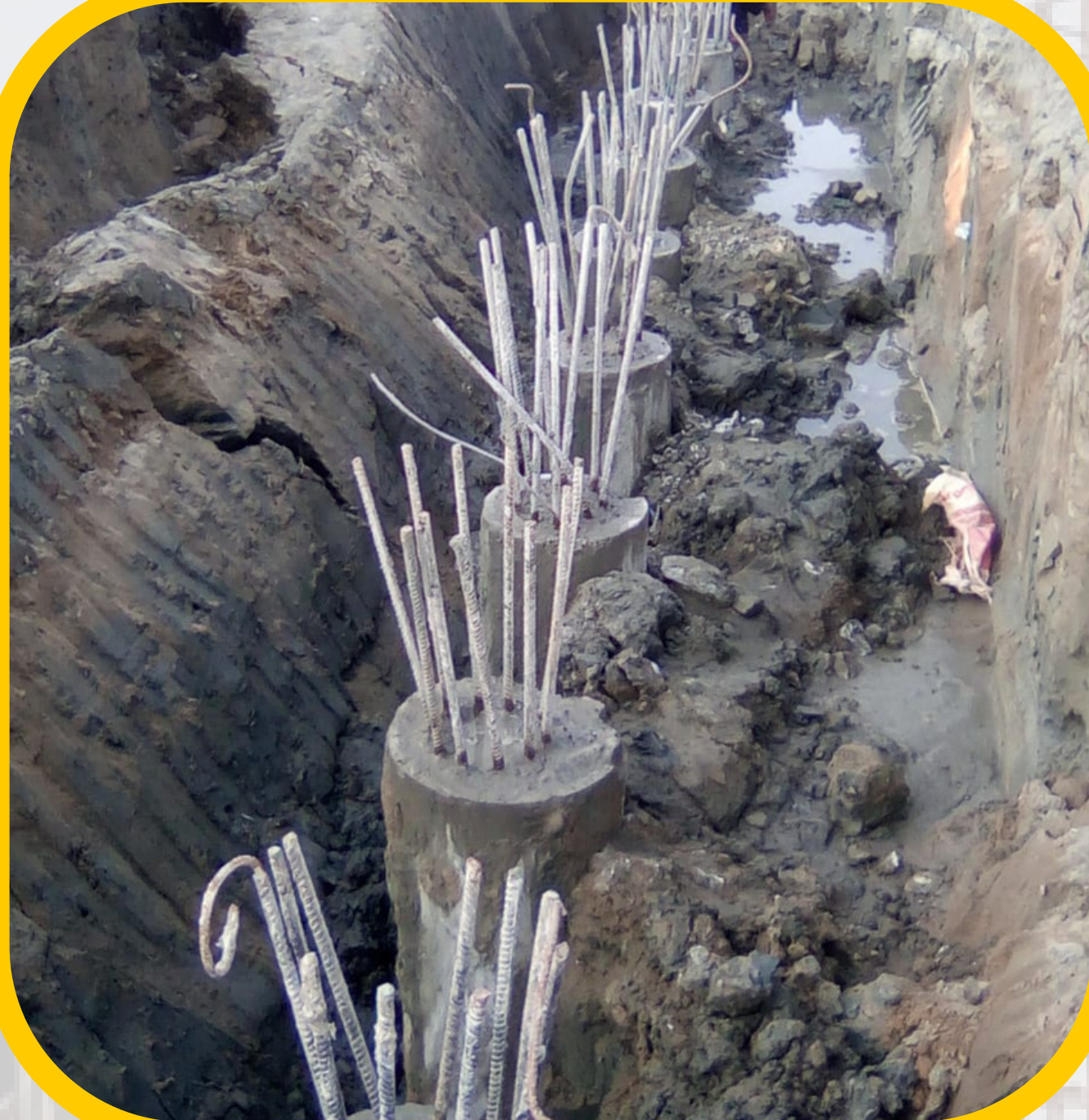
Pile Head Breaking
